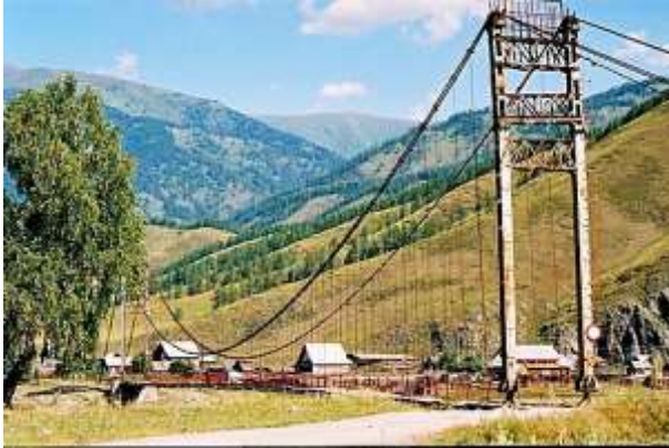
Bridge under Katun river near Tungur village
